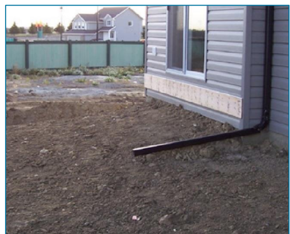
Slope Away From The Foundation Wall
