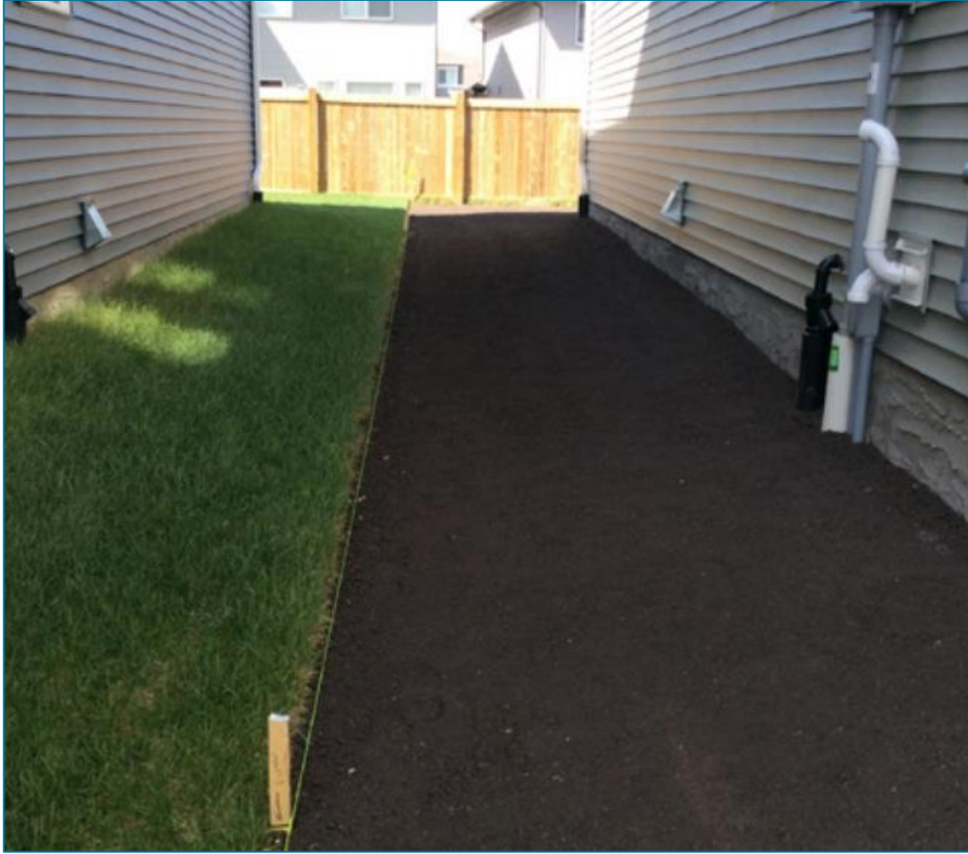
String-line guides used to create consistent minimum 2% slope for drainage swales
