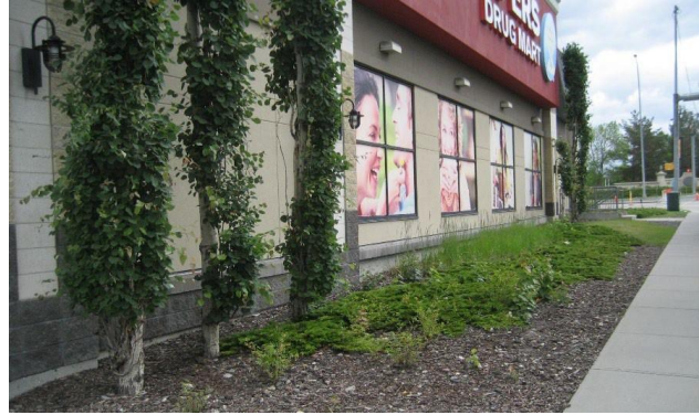
Figure 24: Landscaping and varied exterior materials can provide visual interest on a solid wall and discourage graffiti.
