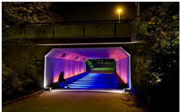
Figure 2: Attractive, even lighting, and clear sightlines help make this pedestrian underpass feel safer after dark. (Image: CITYSPOT)
