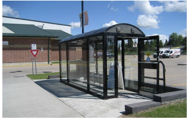
Figure 3: The transit stop at Ken Nichol Regional Recreation Centre incorporates a transparent, weatherproof, well-lit shelter in a location that is visible from the street and the Centre entrance.
