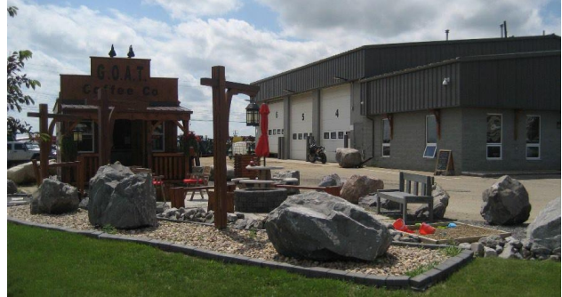
Figure 29 A small-scale, locally owned coffee shop on a visible corner offers a gathering place within an industrial area and supports capacity, culture, and cohesion.
