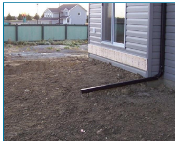
Slope Away From The Foundation Wall
