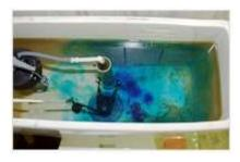
Wait 15-30 minutes. If the water in the toilet bowl changes colors, the flapper valve needs to be replaced. The flapper valve is located at the bottom of the tank; flapper valve kits are available at most hardware and home supply stores.
