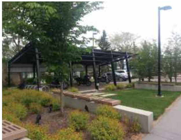
Architectural screening and plantings help to reduce the impact of parking areas without compromising views into those areas.
