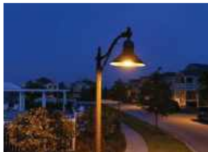
Dark sky fixtures shield the light bulb and direct light downward to limit light pollution.
