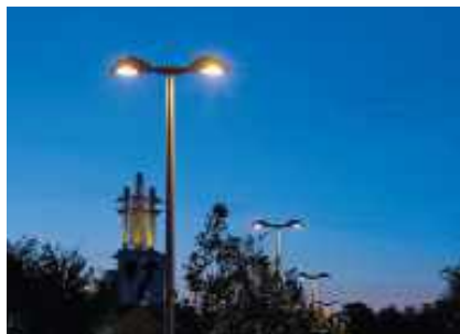
Dark sky fixtures shield the light bulb and direct light downward to limit light pollution.
