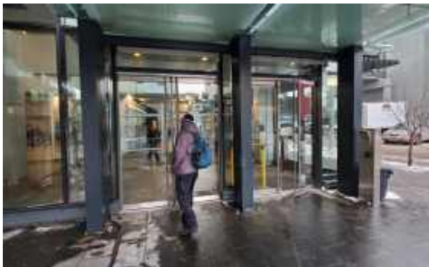
Vestibules at building entrances prevent heat loss for buildings.
