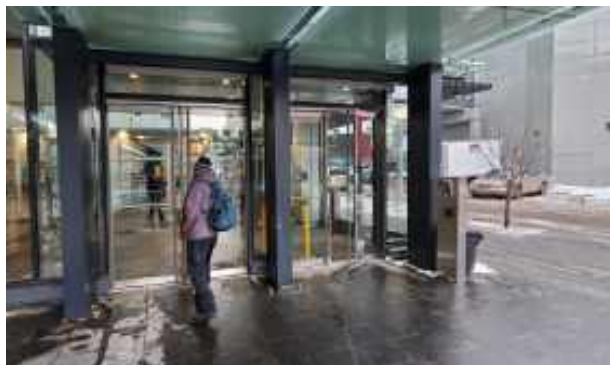
Vestibules can be provided at building entrances to help prevent heat loss from the building.
