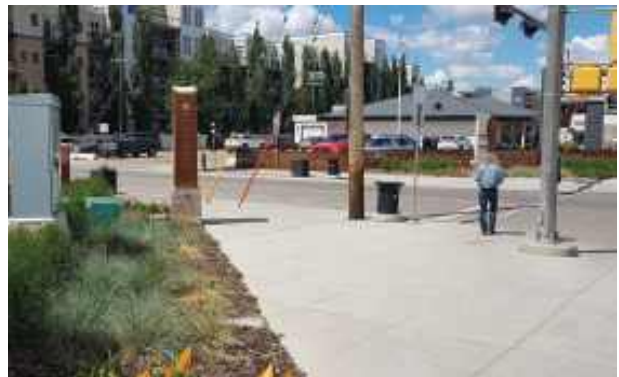
Utility boxes are screened from view and integrated into landscaping in this section of 105 th Avenue in Edmonton.
