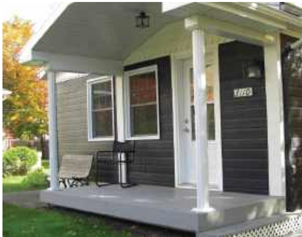
House with exterior porch at grade.
