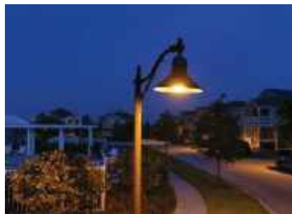
Dark sky fixtures shield the light bulb and direct light downward
