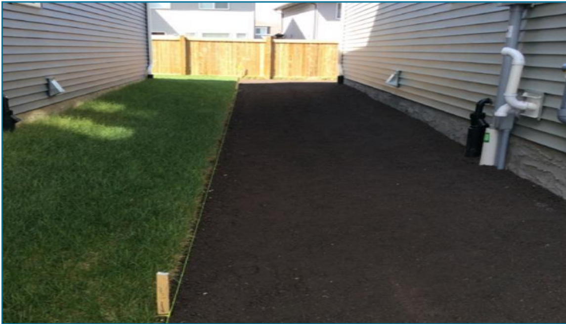
String-line guides used to create consistent minimum 2% slope for drainage swale
