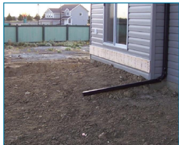
Slope Away From The Foundation Wall
