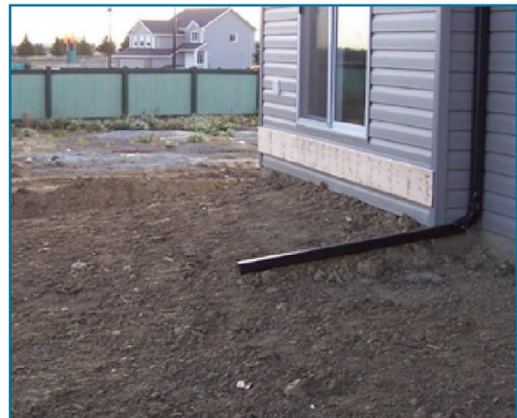
Slope Away From The Foundation Wall
