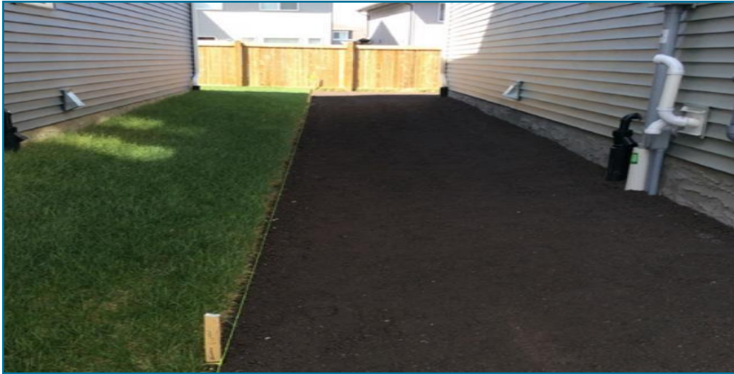
String-line guides used to create consistent minimum 2% slope for drainage swale
